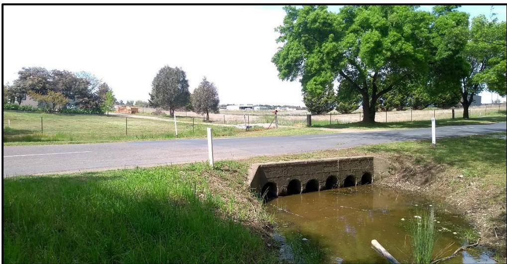
Plate 2 - Floodway from the Site discharging through a multi-pipe culvert at Green Street. Southern view towards the Site.
